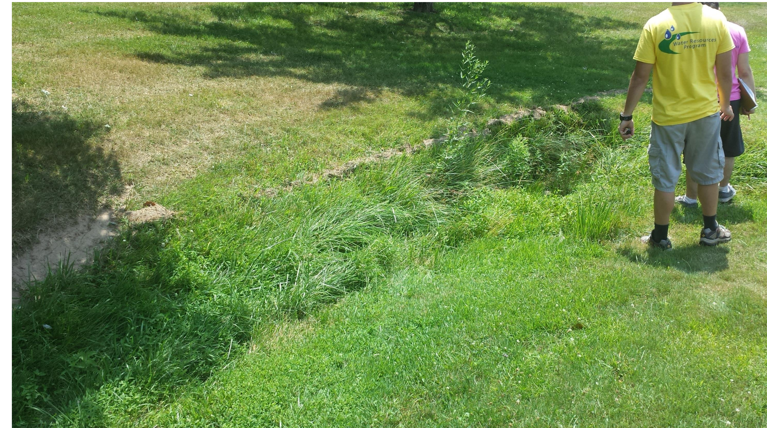
Swale feature leading to basin
