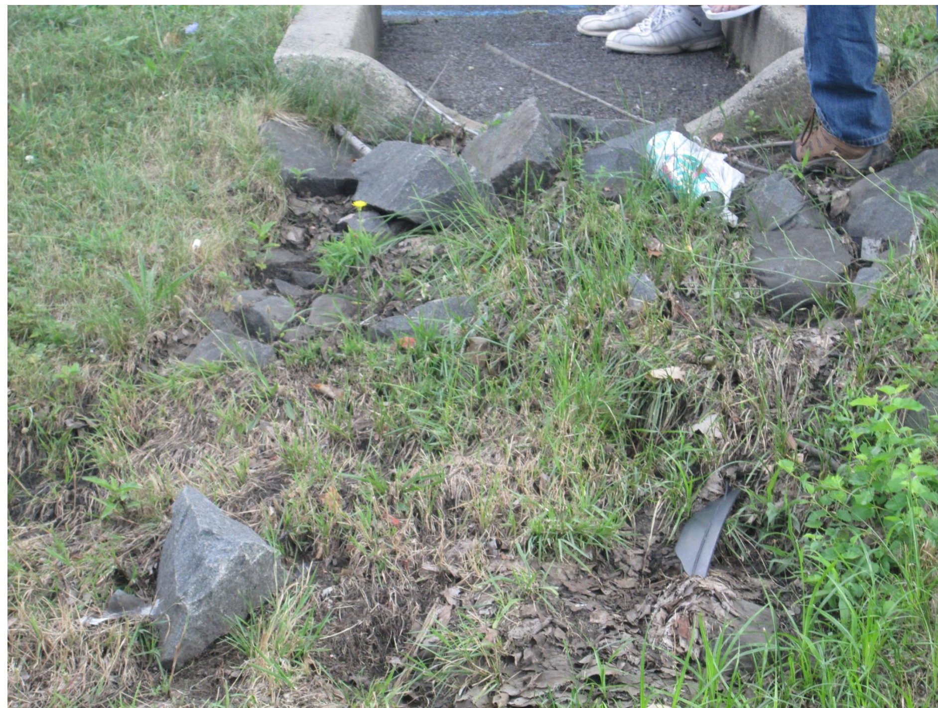
Curb-cut from parking lot
