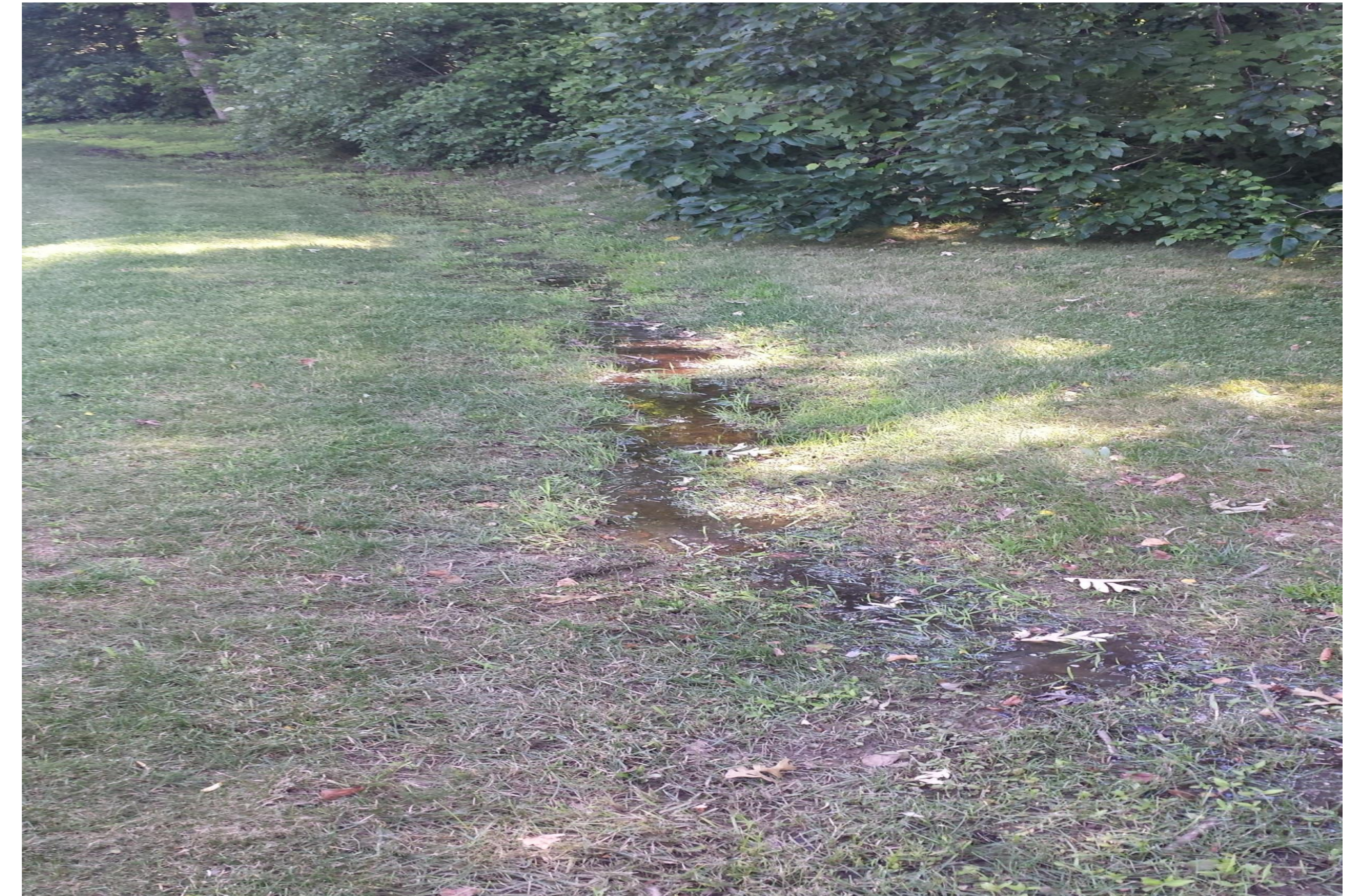
Swale exiting basin
