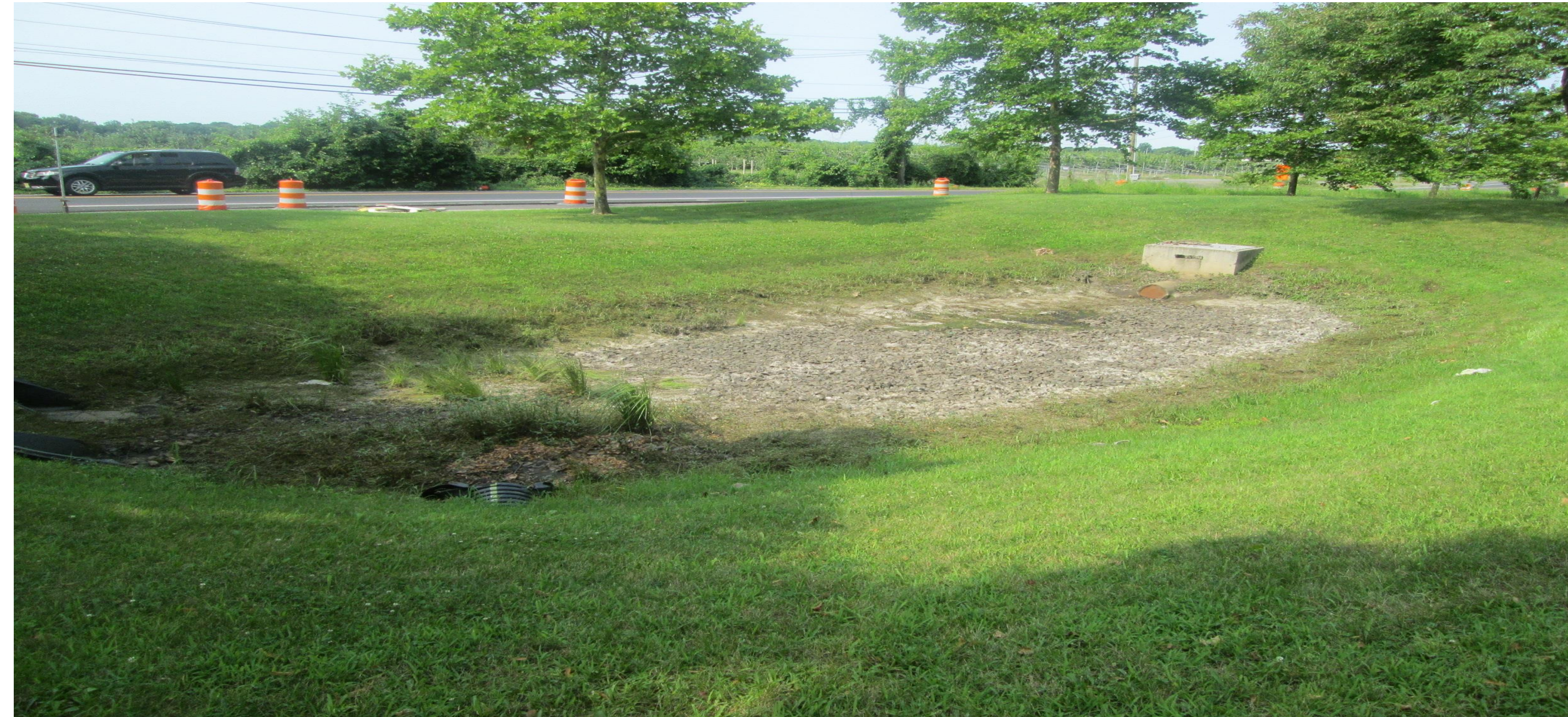
Overview of basin
