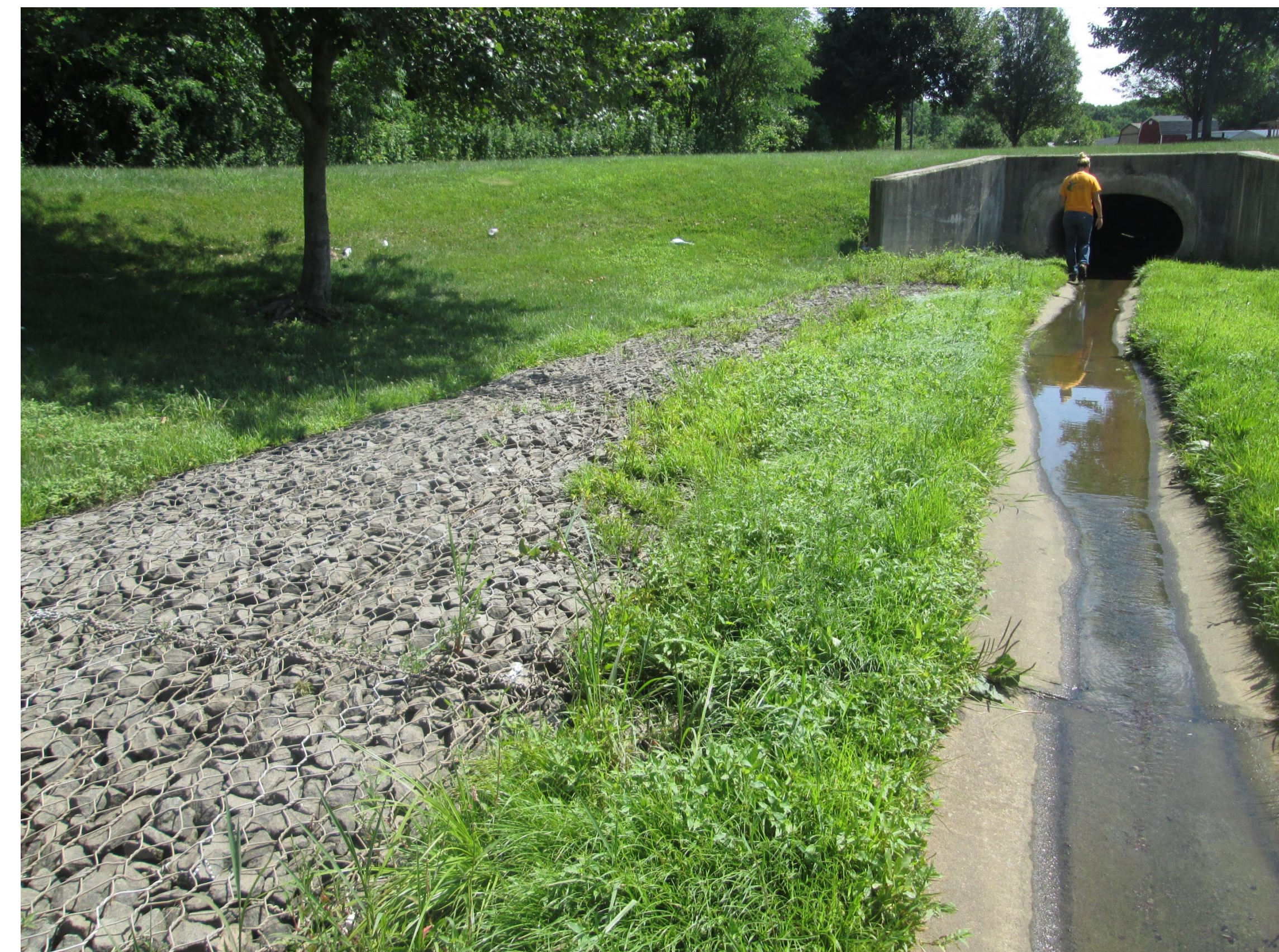
Rip-rap by inlet
