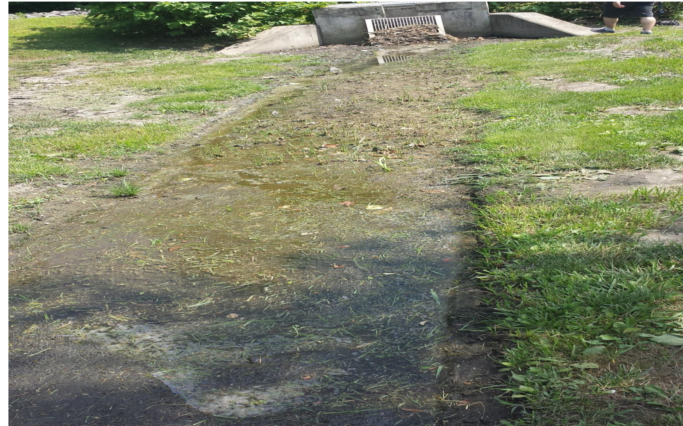
Low flow channel leading to outlet
