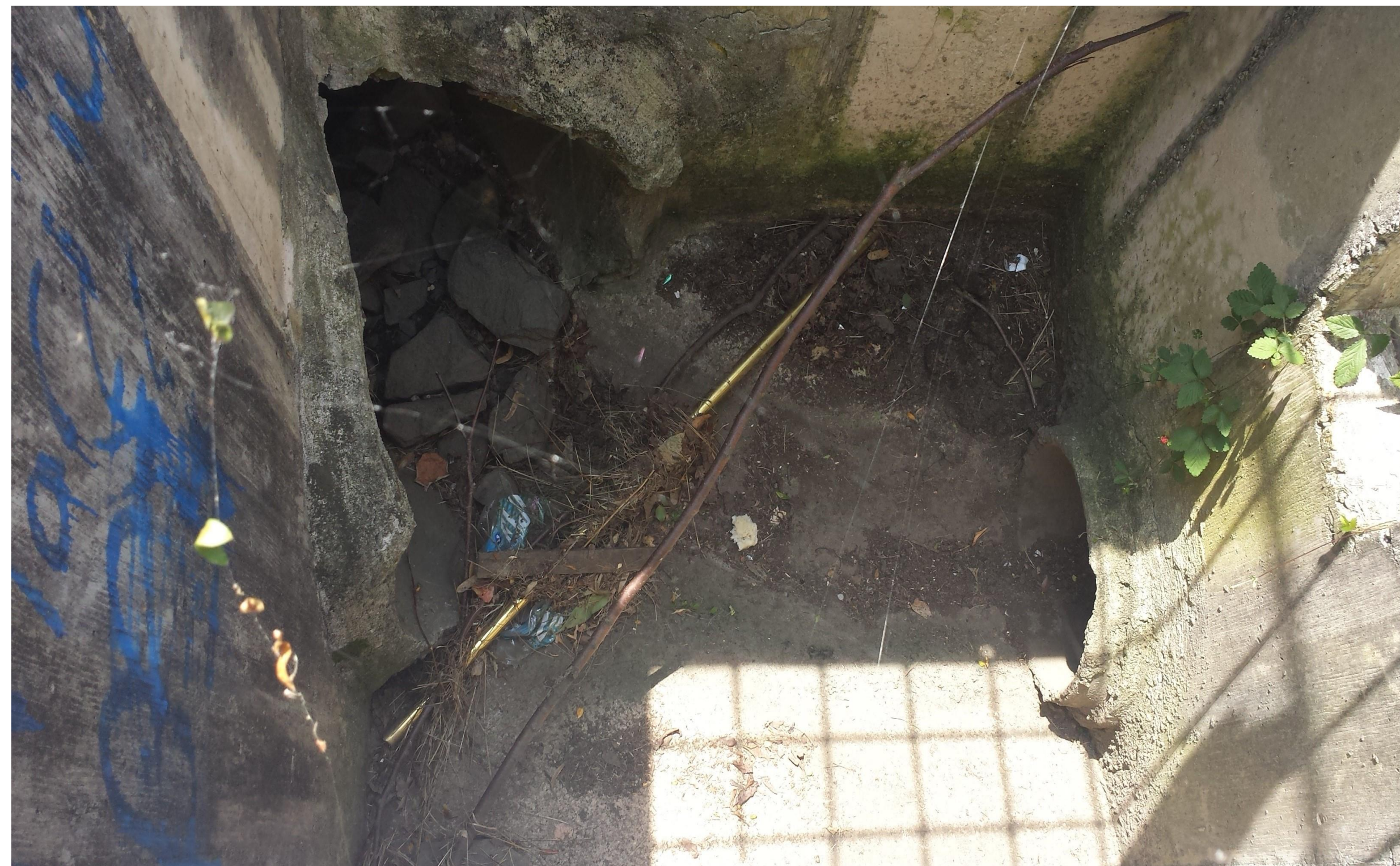
Inside of outlet
