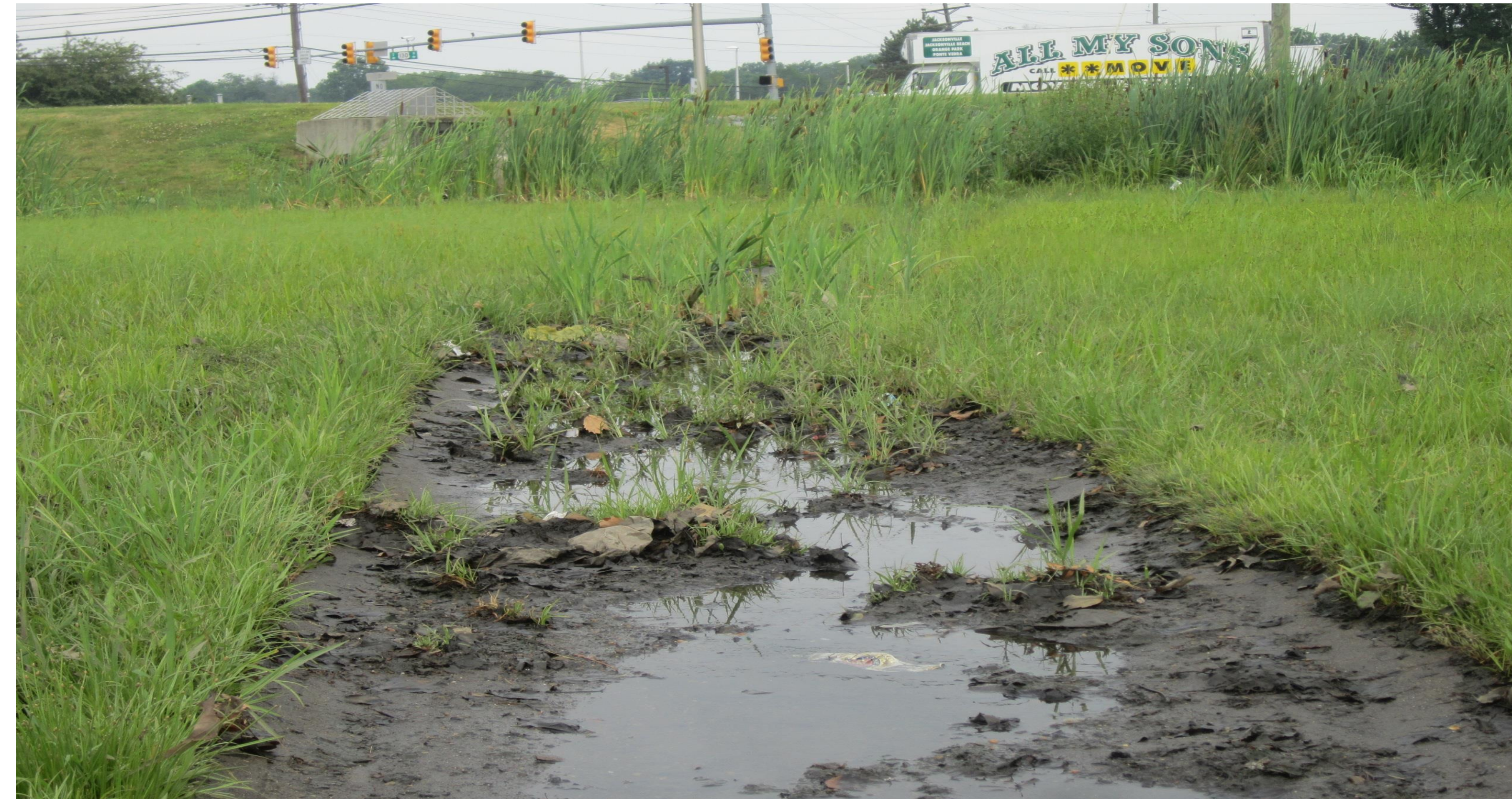
Sediment accumulation
