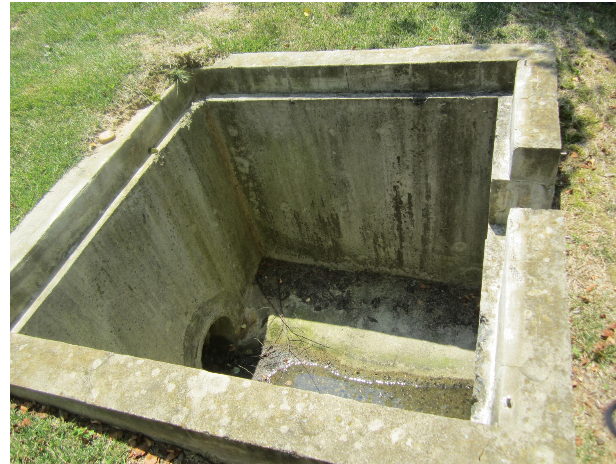
Top view of outlet structure
