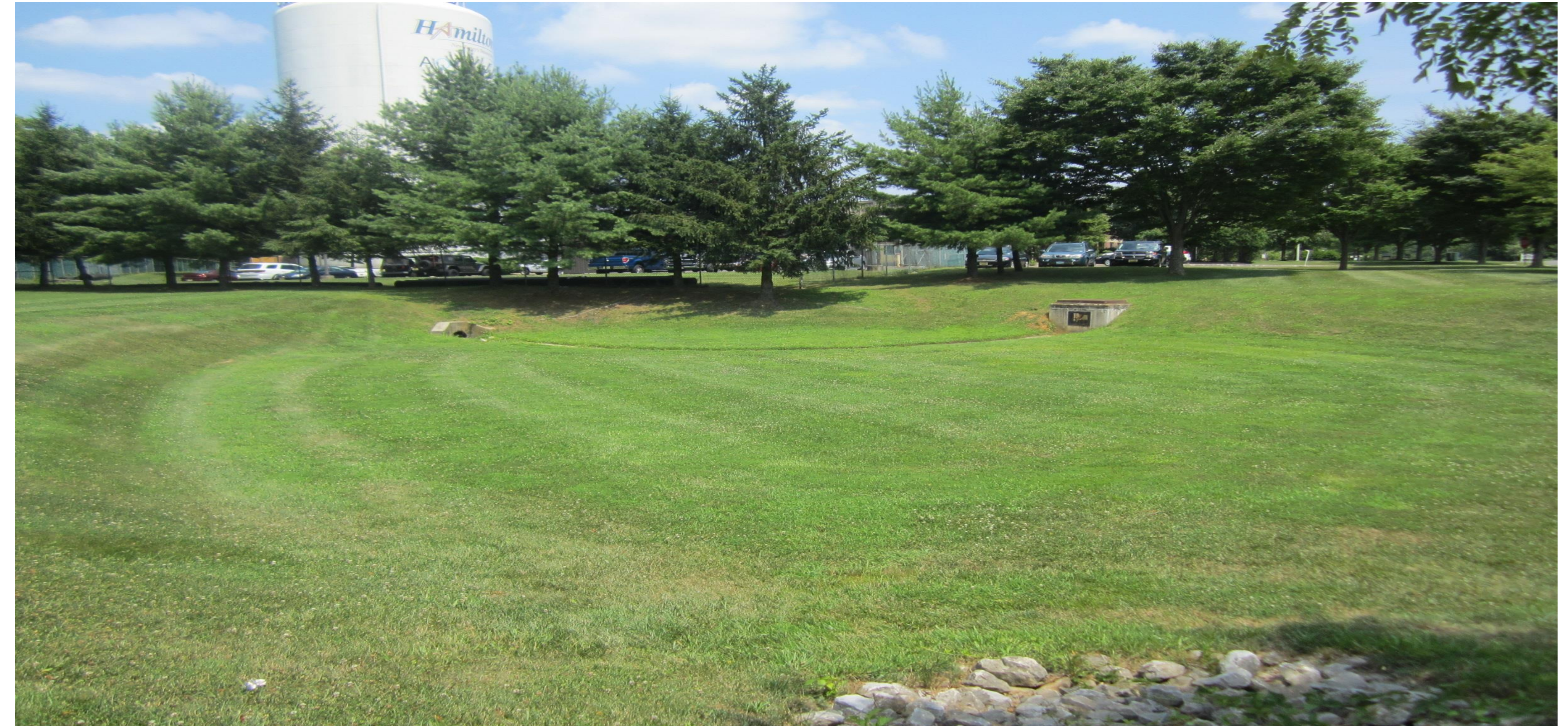
Overview of basin
