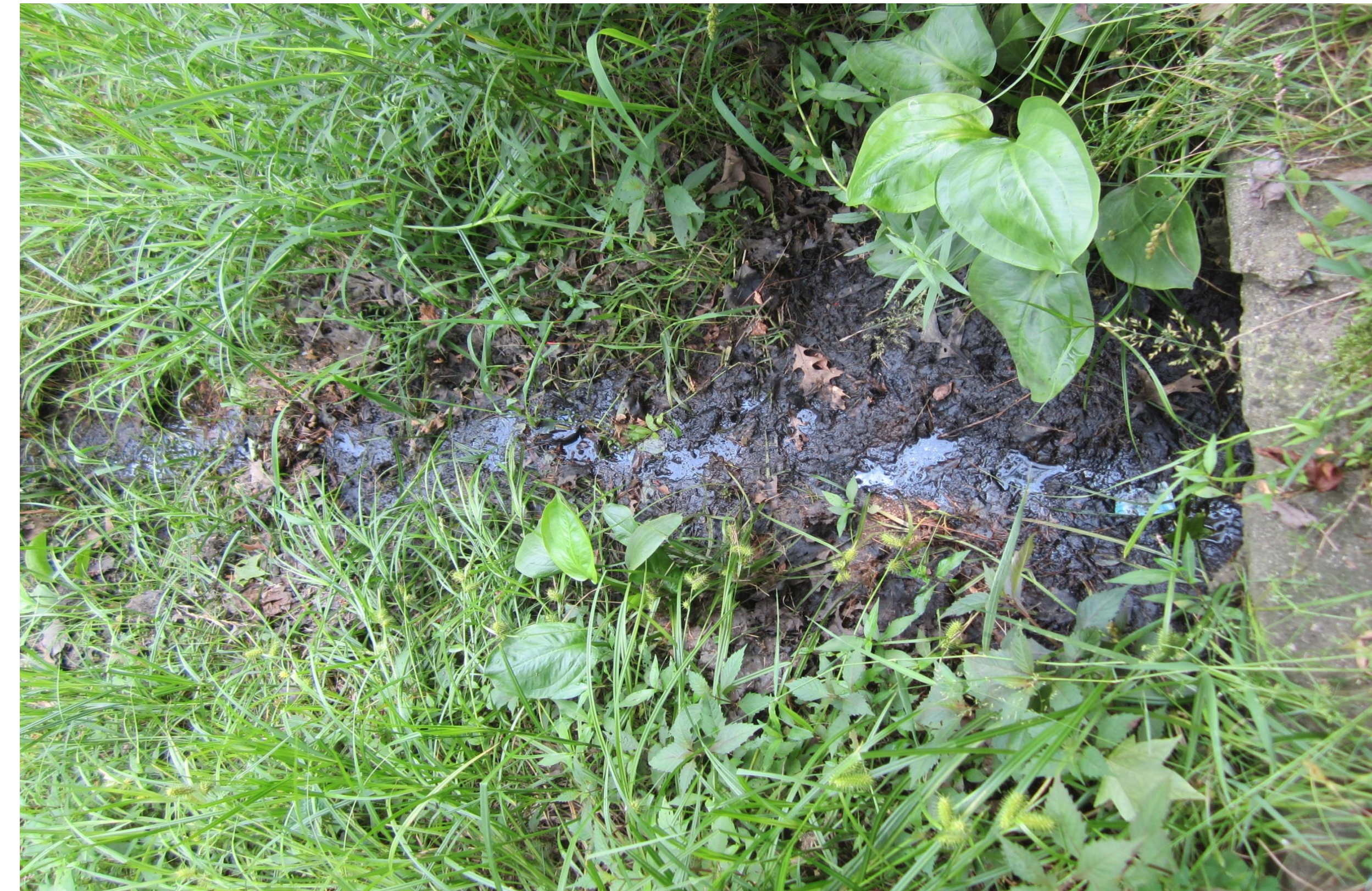
Low flow channel near outlet
