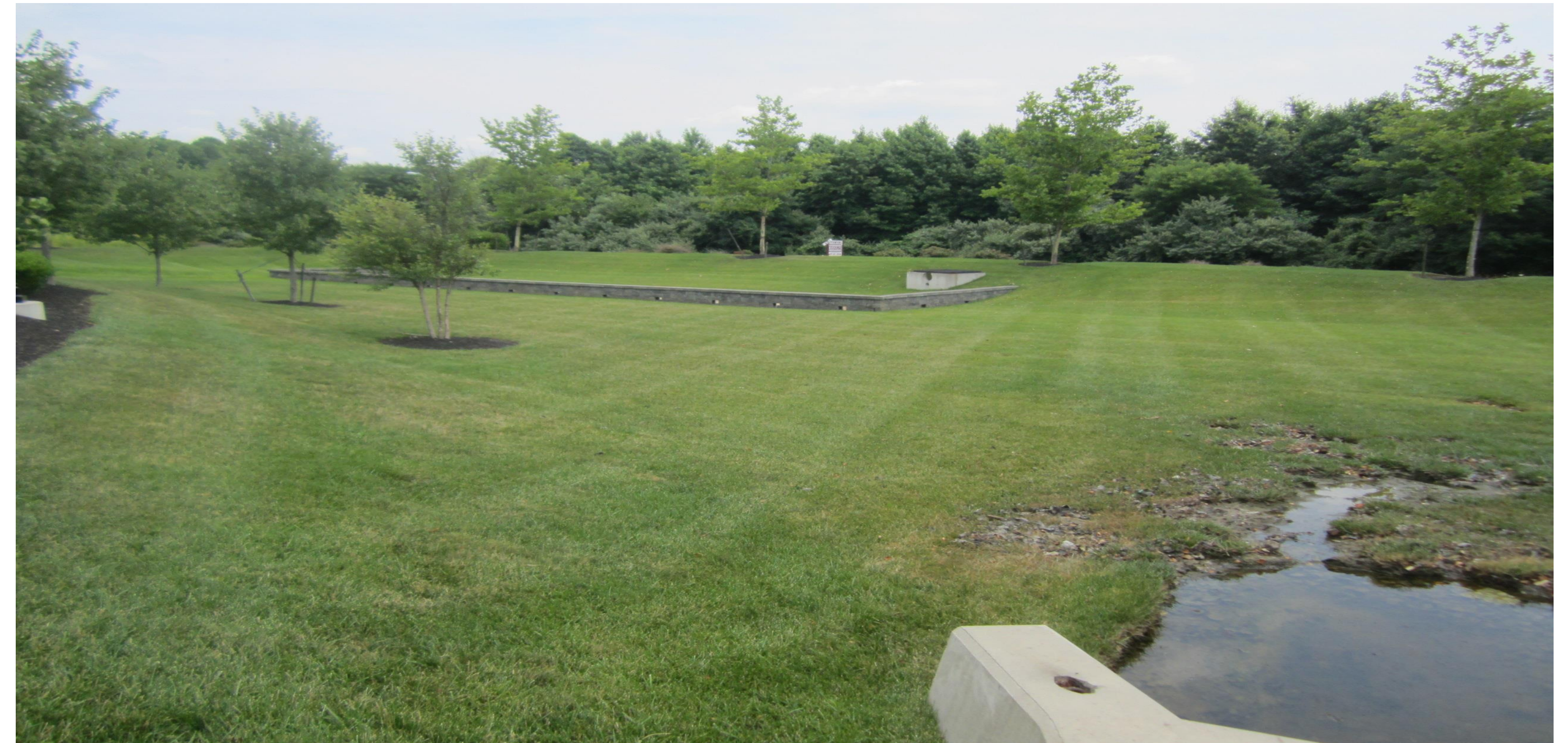
Overview of basin
