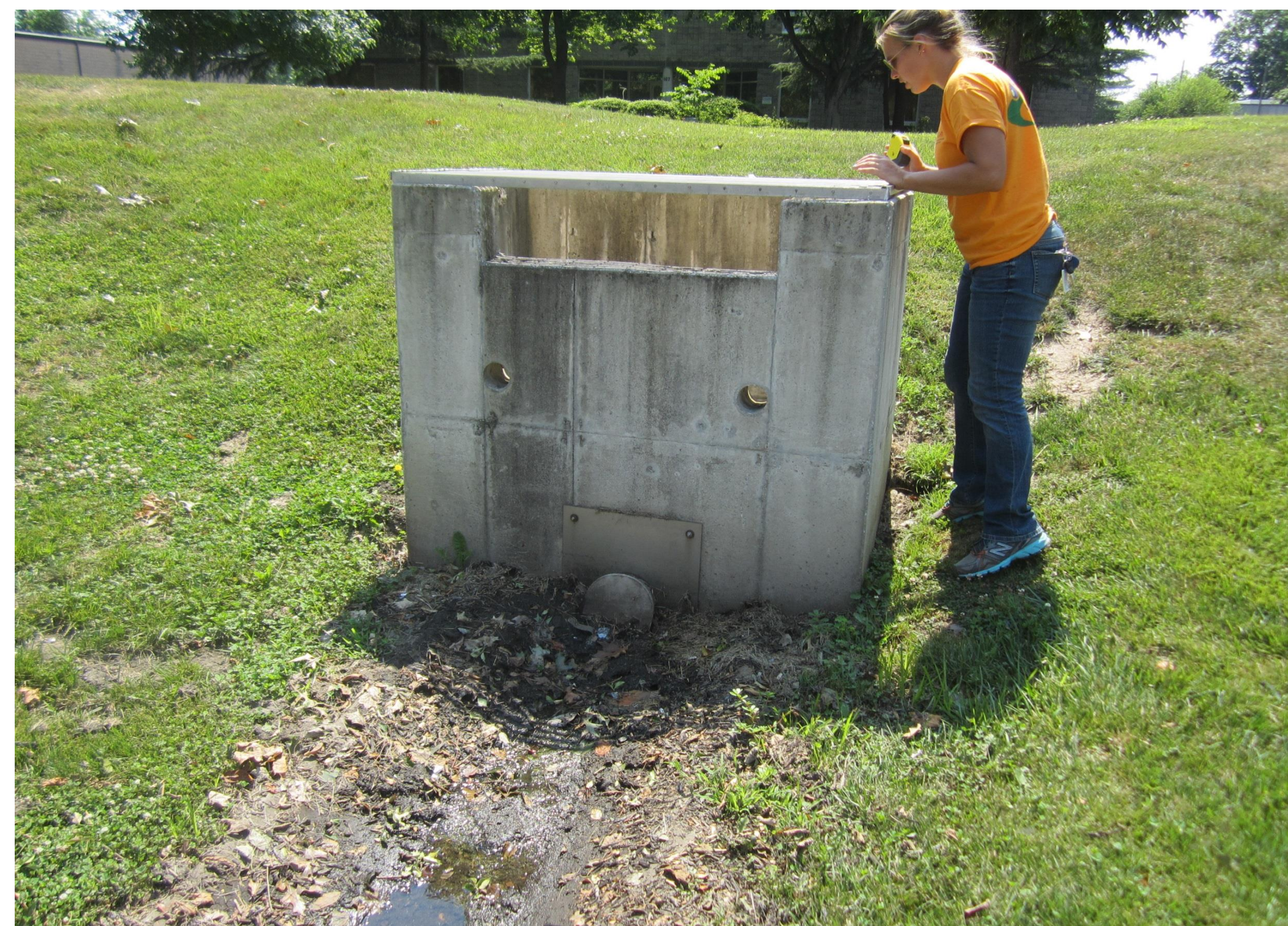
Front view of outlet structure
