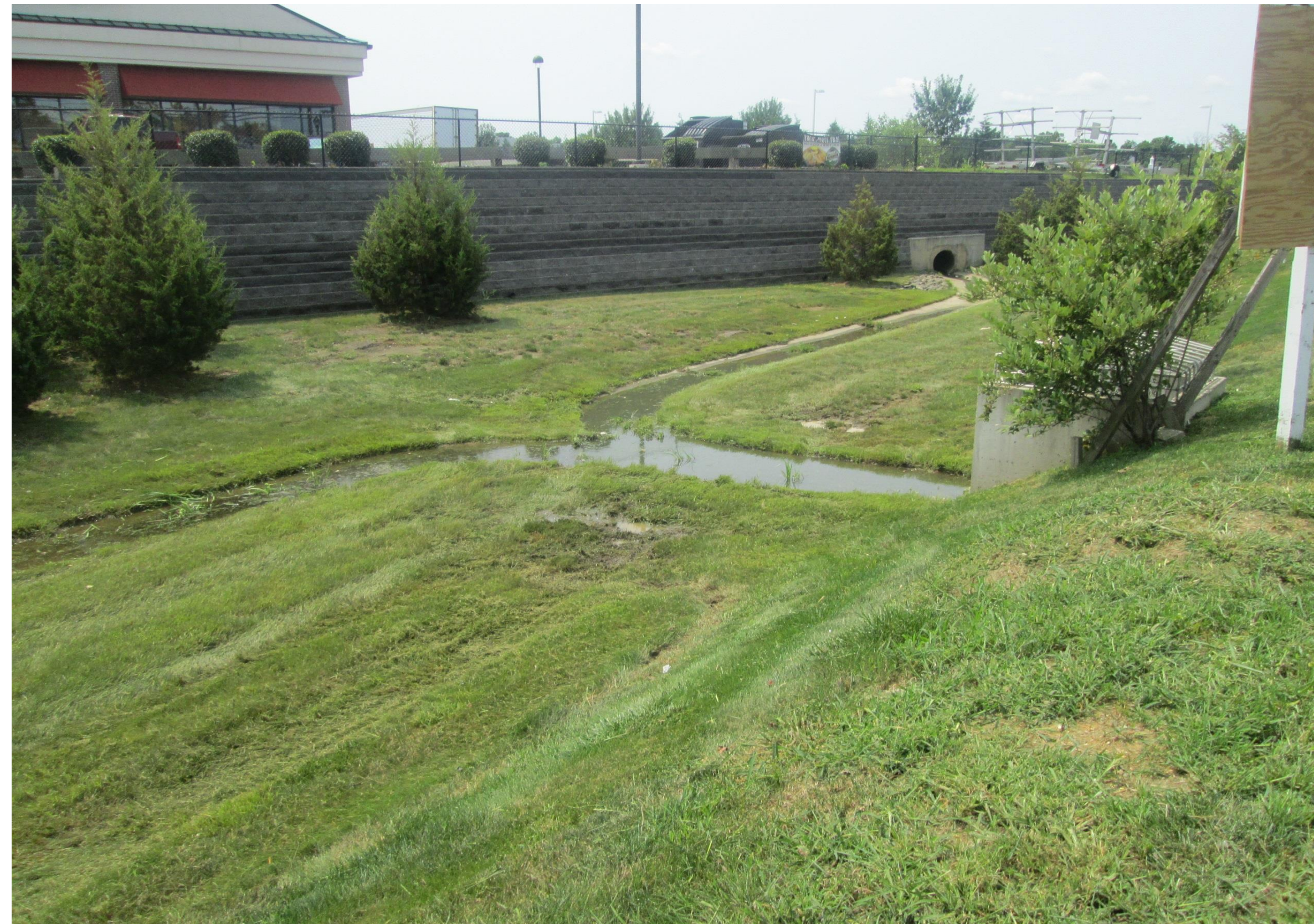
Overview of basin
