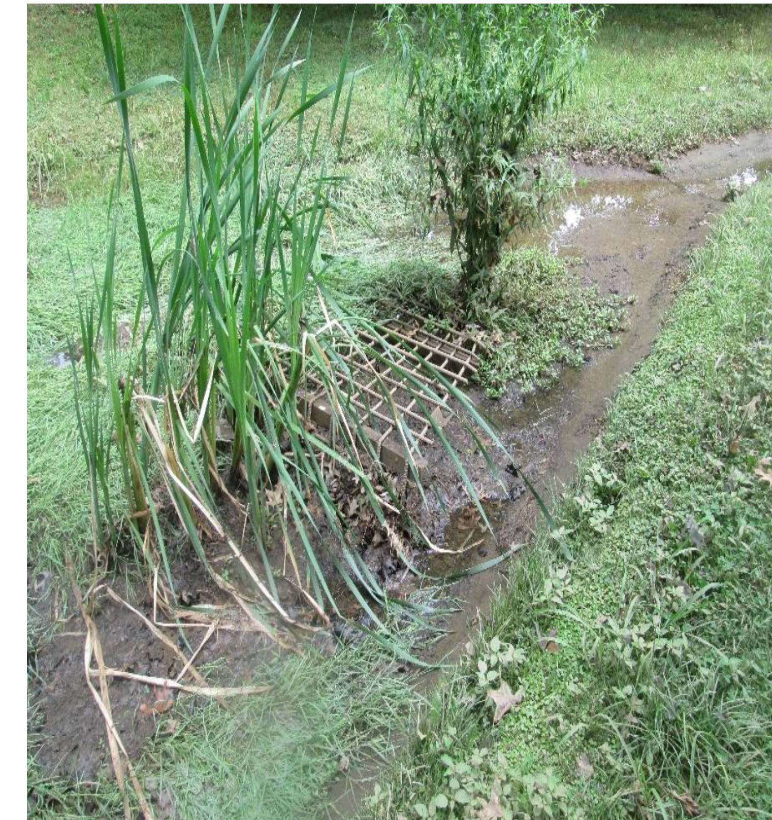
Metal grate in low flow channel
