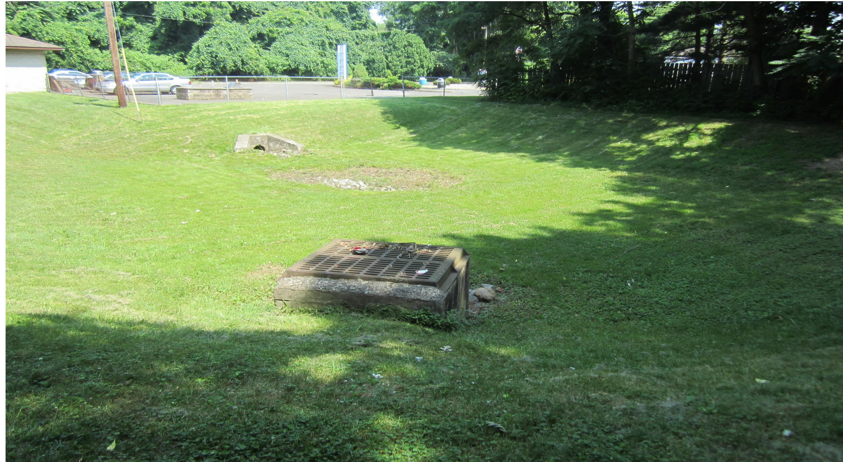
Overview of basin
