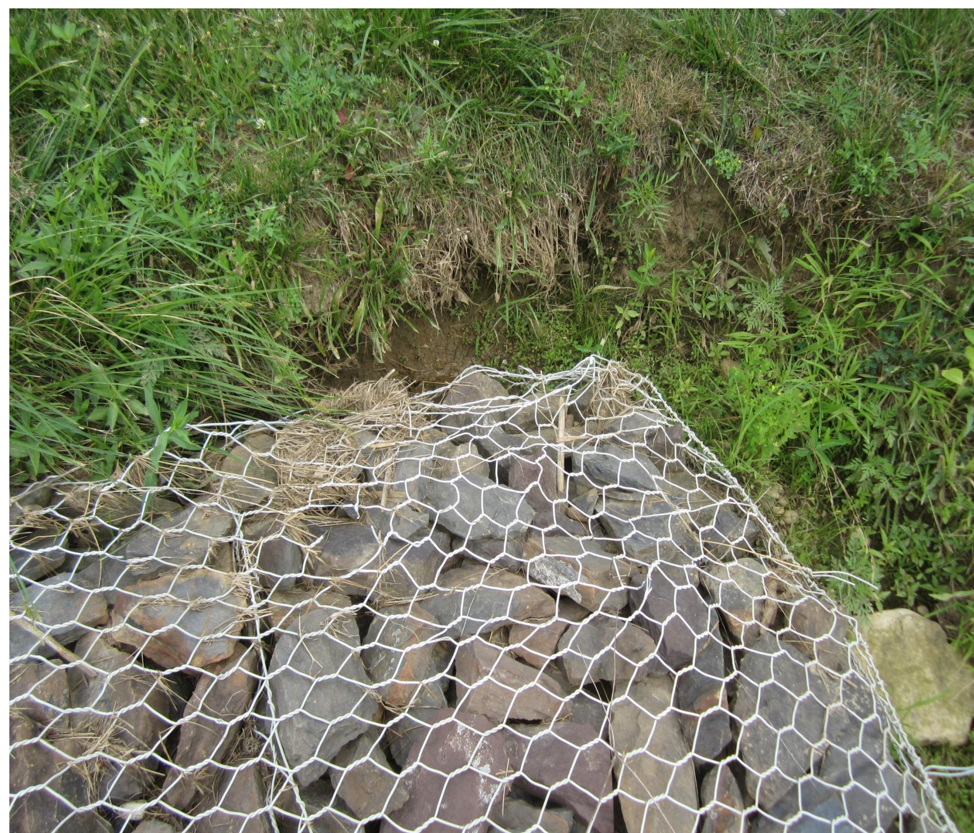
Eroded embankment
