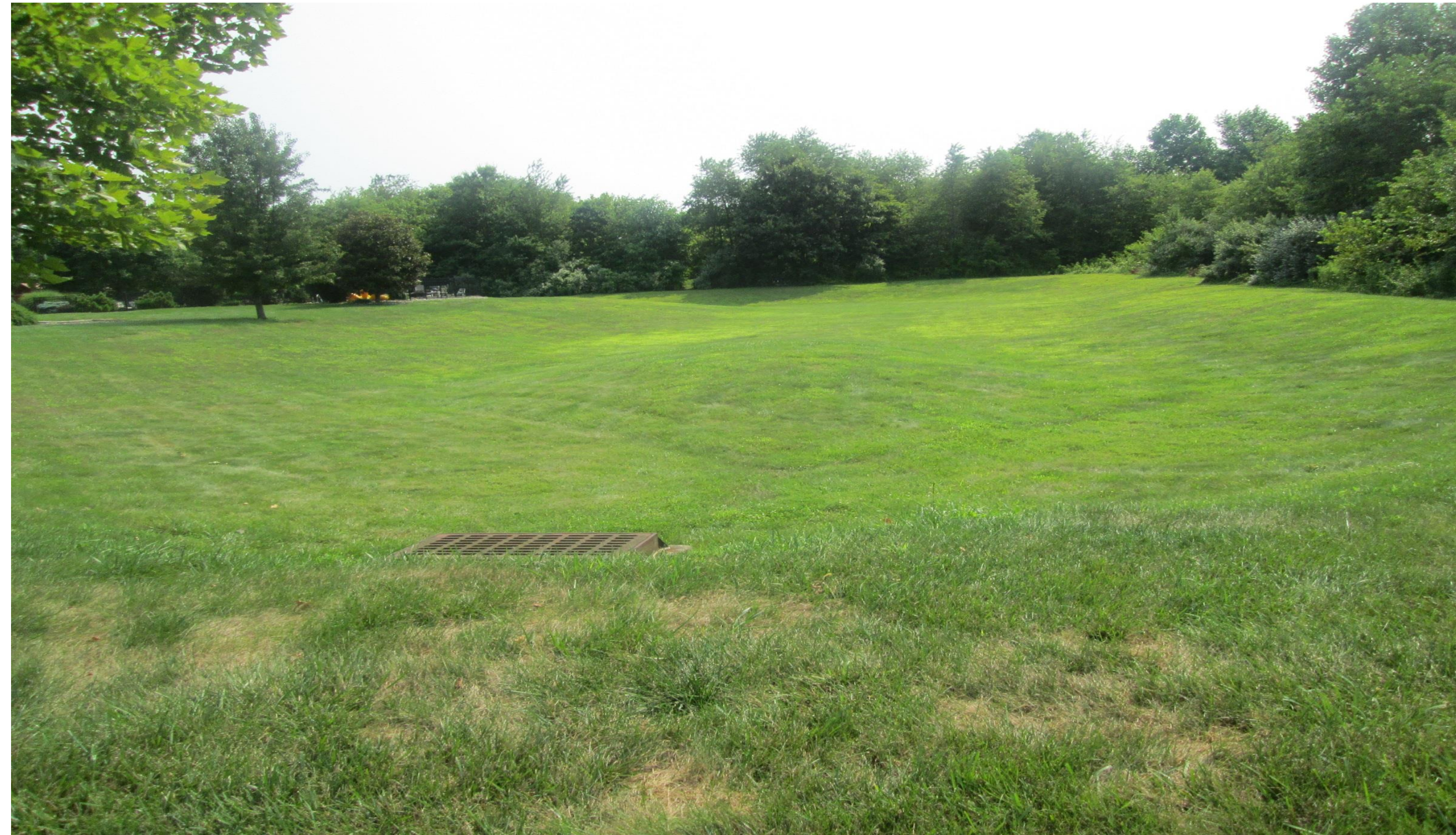
Overview of basin
