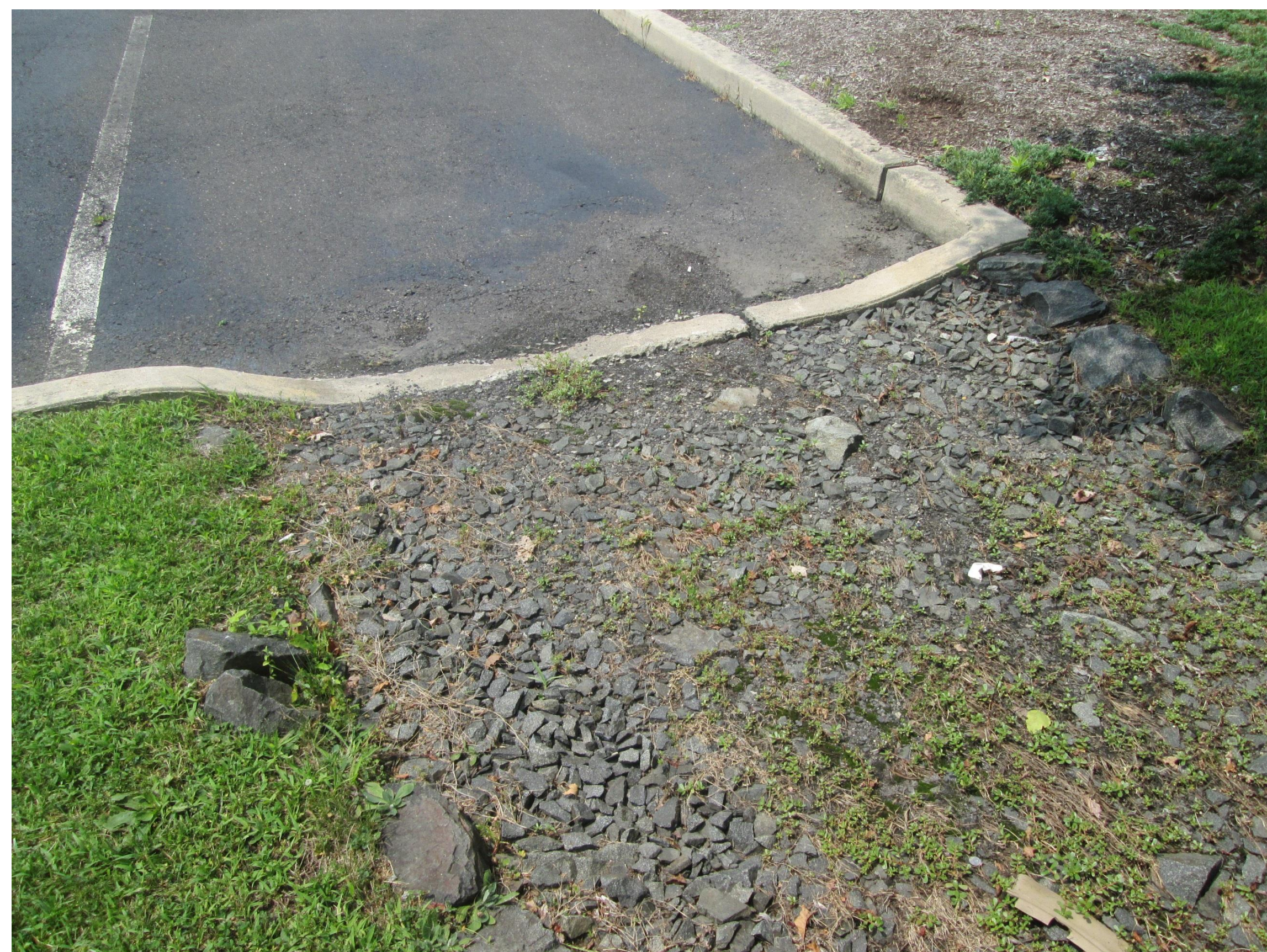
Curb-cut leading to basin
