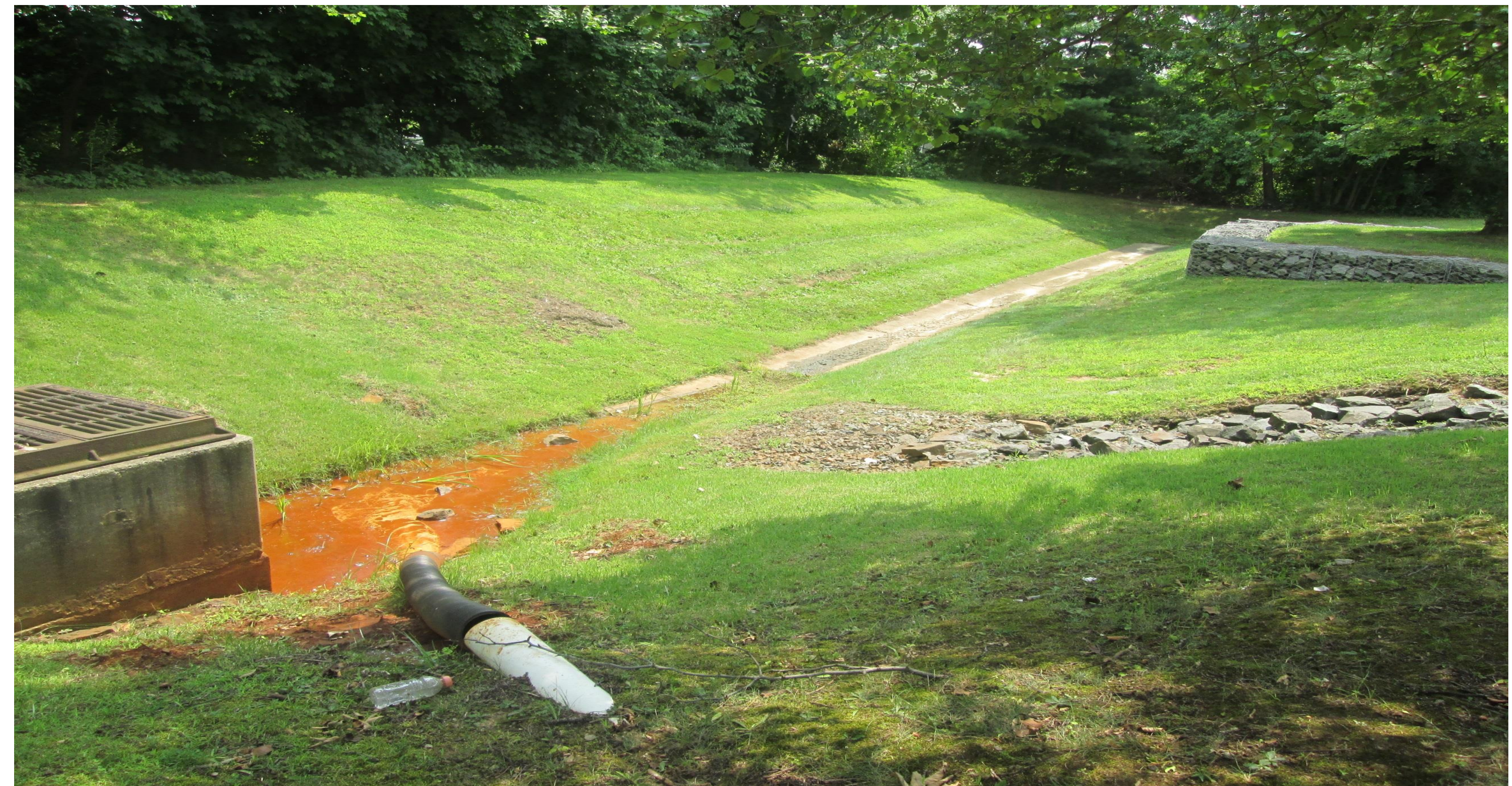
Overview of basin
