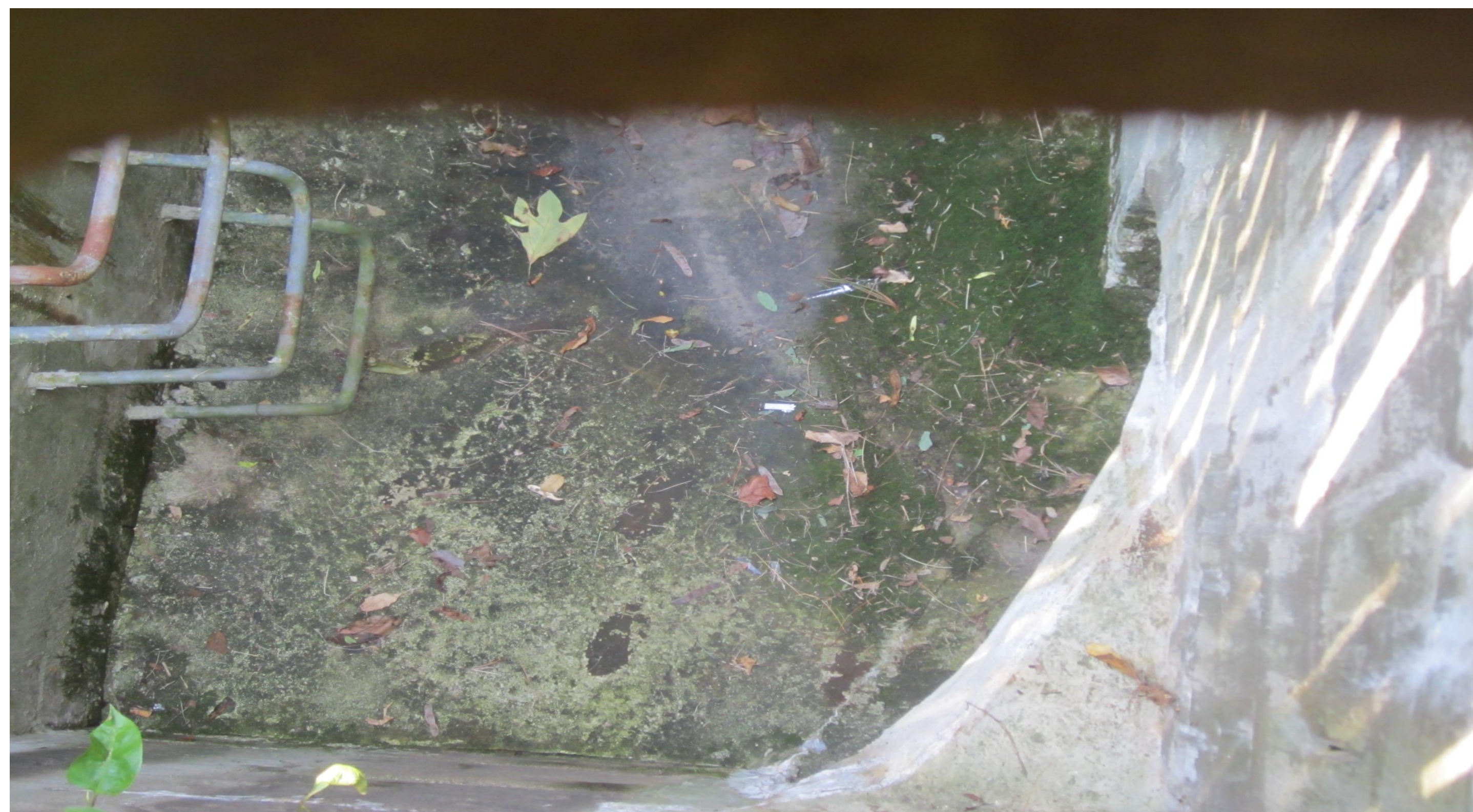
Inside of outlet
