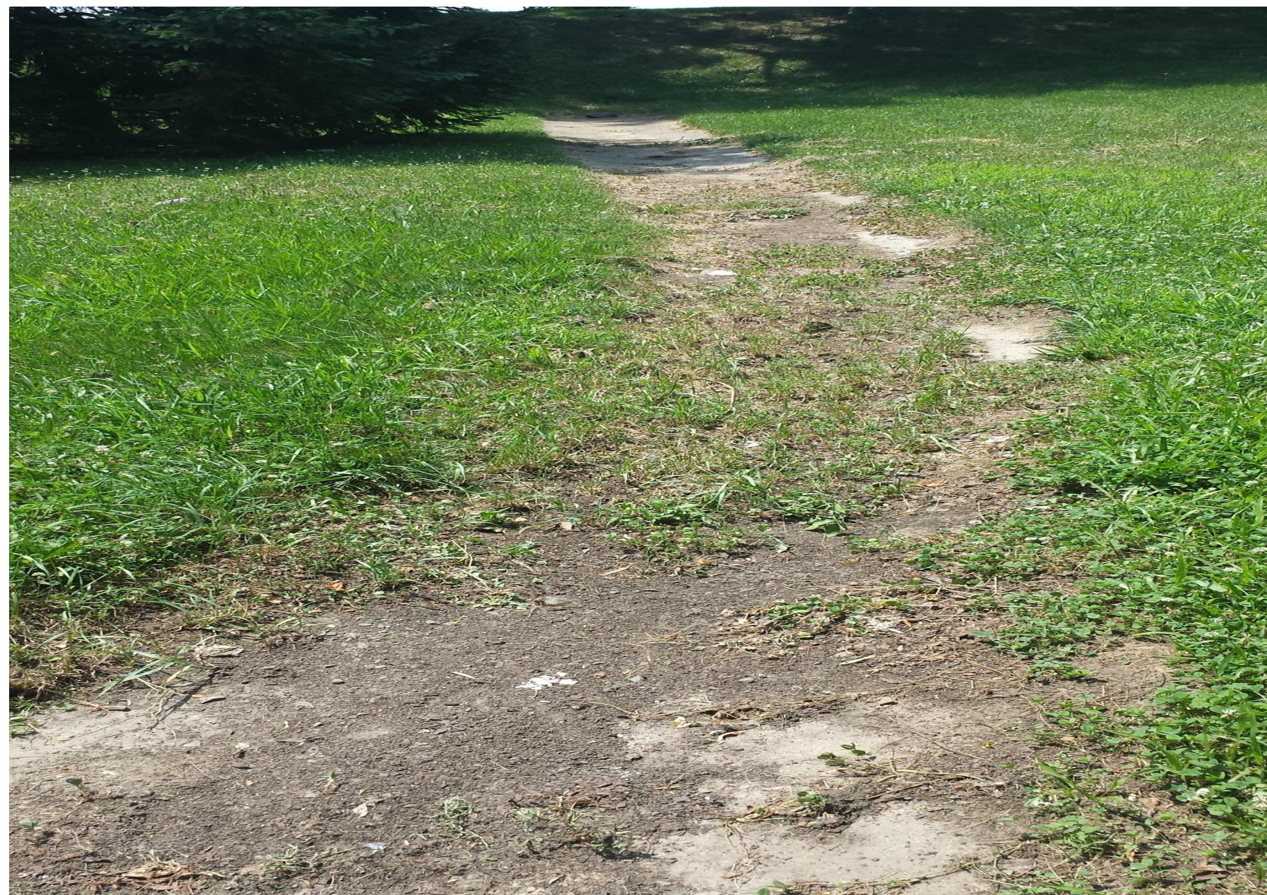
Overgrown on low flow channel
