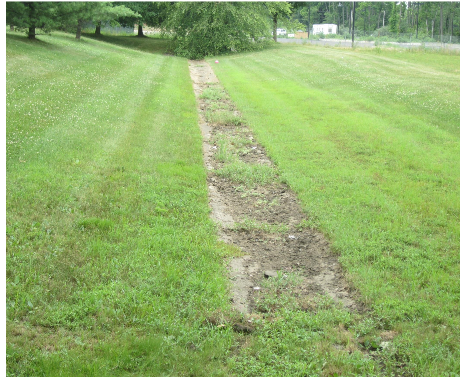
Sediment in low flow channel
