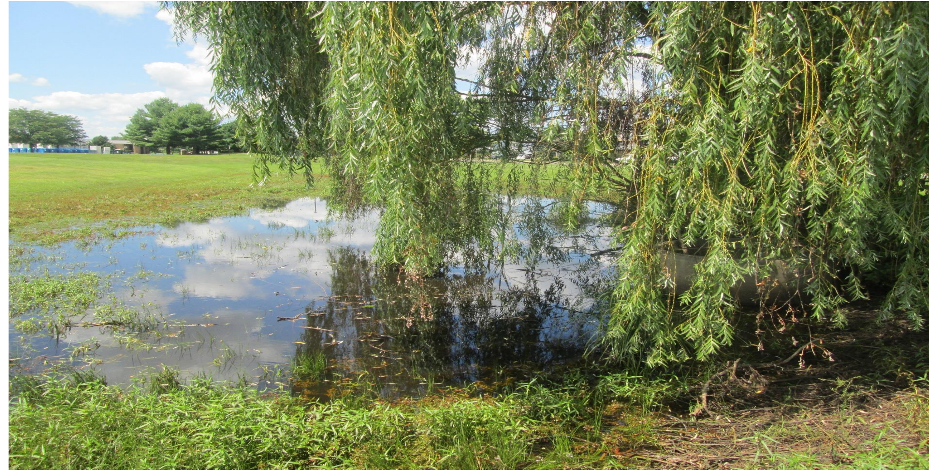
Overview of Basin
