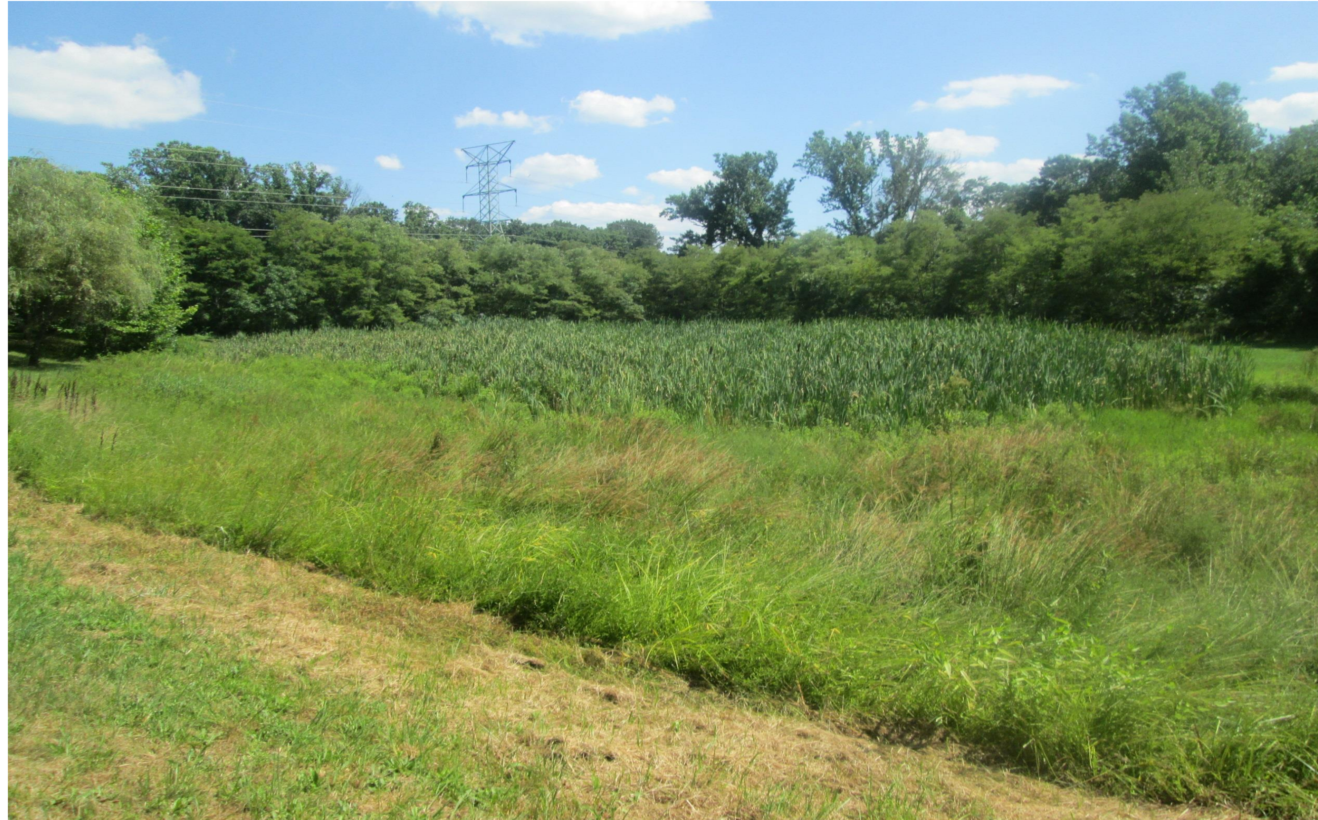
Overview of basin
