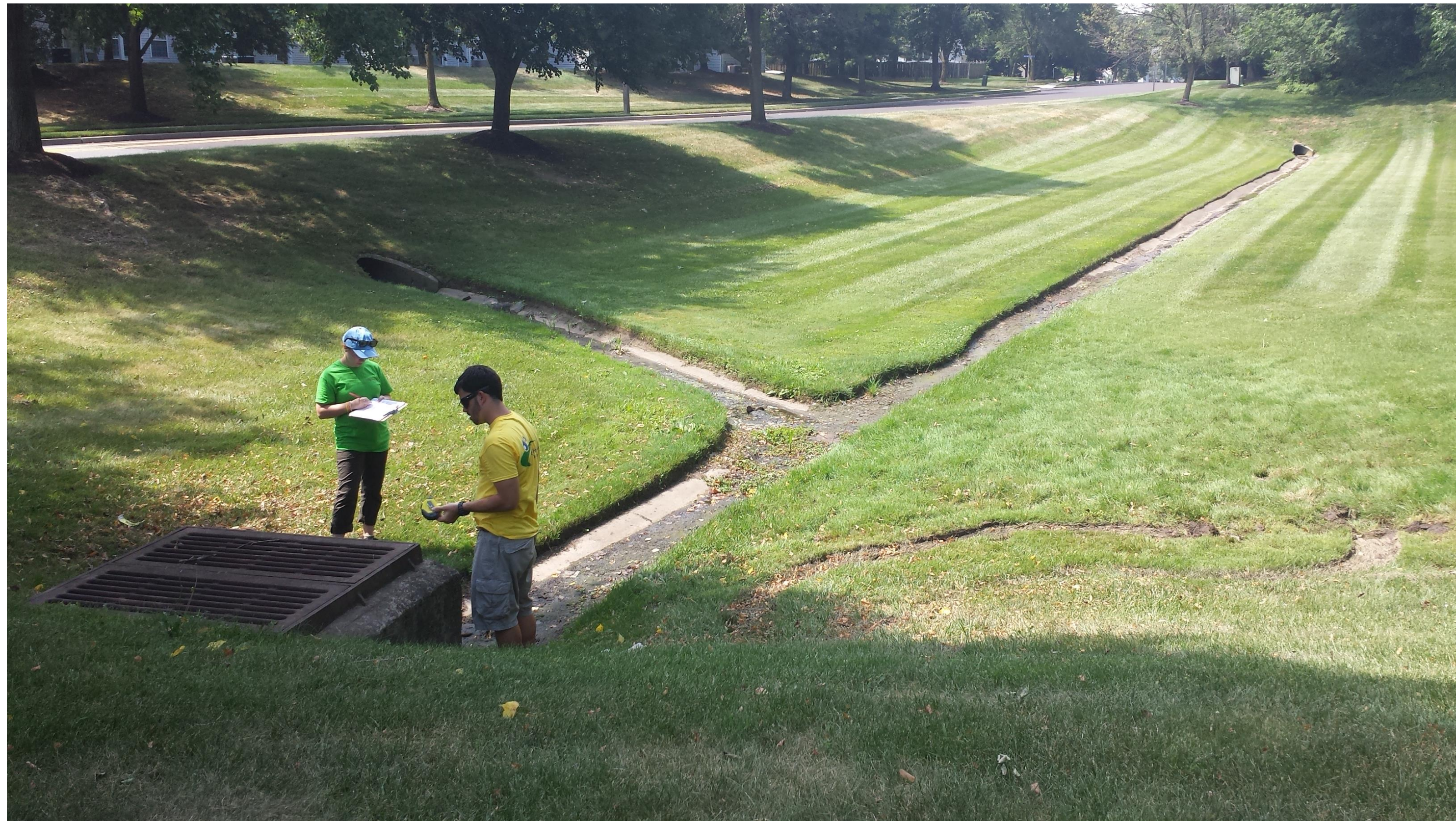
Overview of basin
