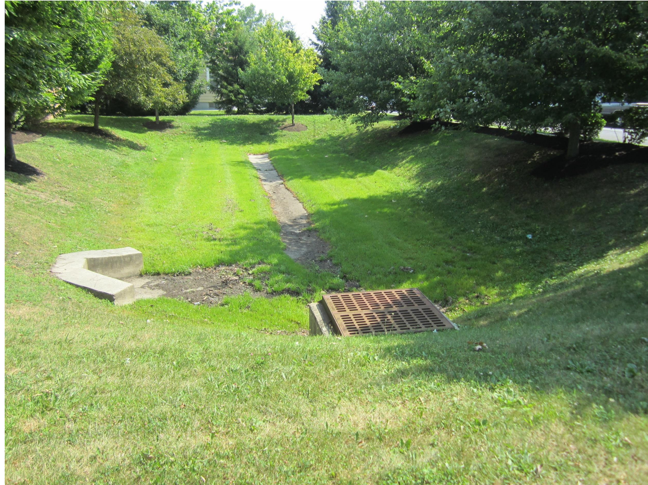
Overview of basin
