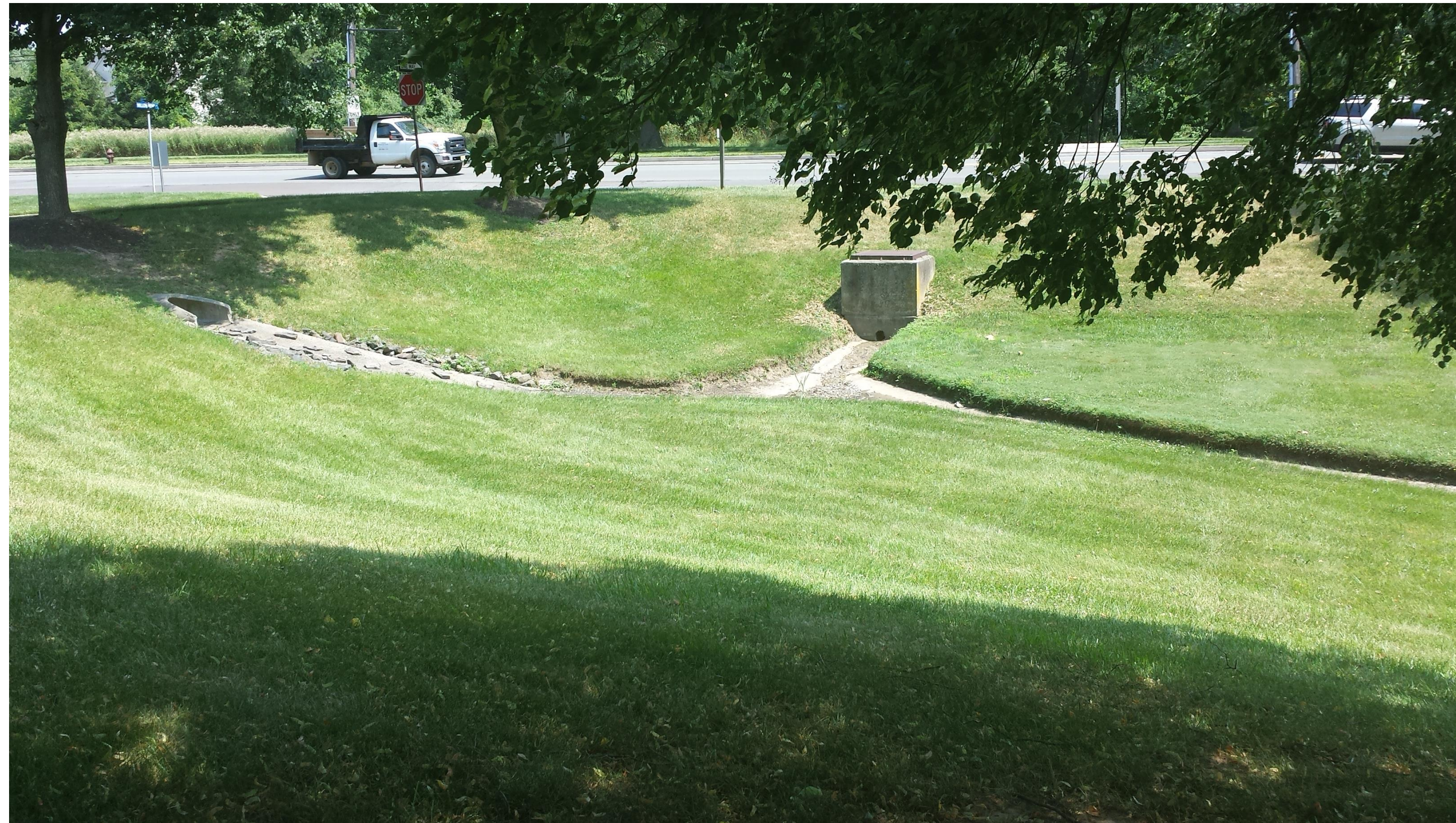
Overview of basin
