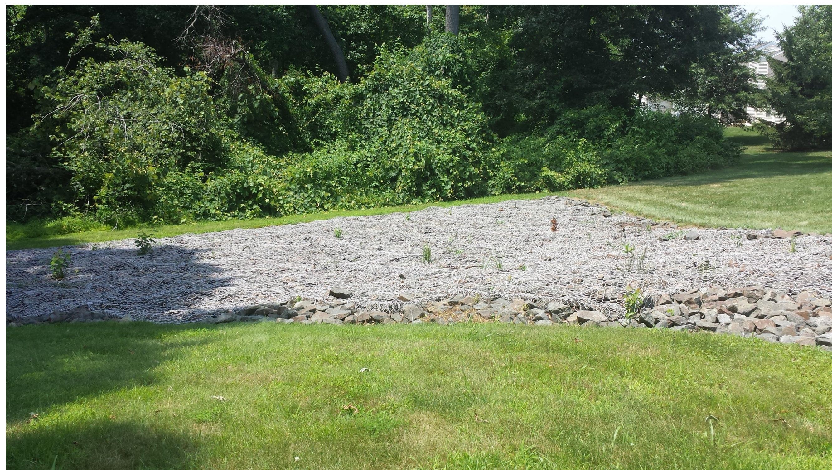
Stone bed as emergency spillway
