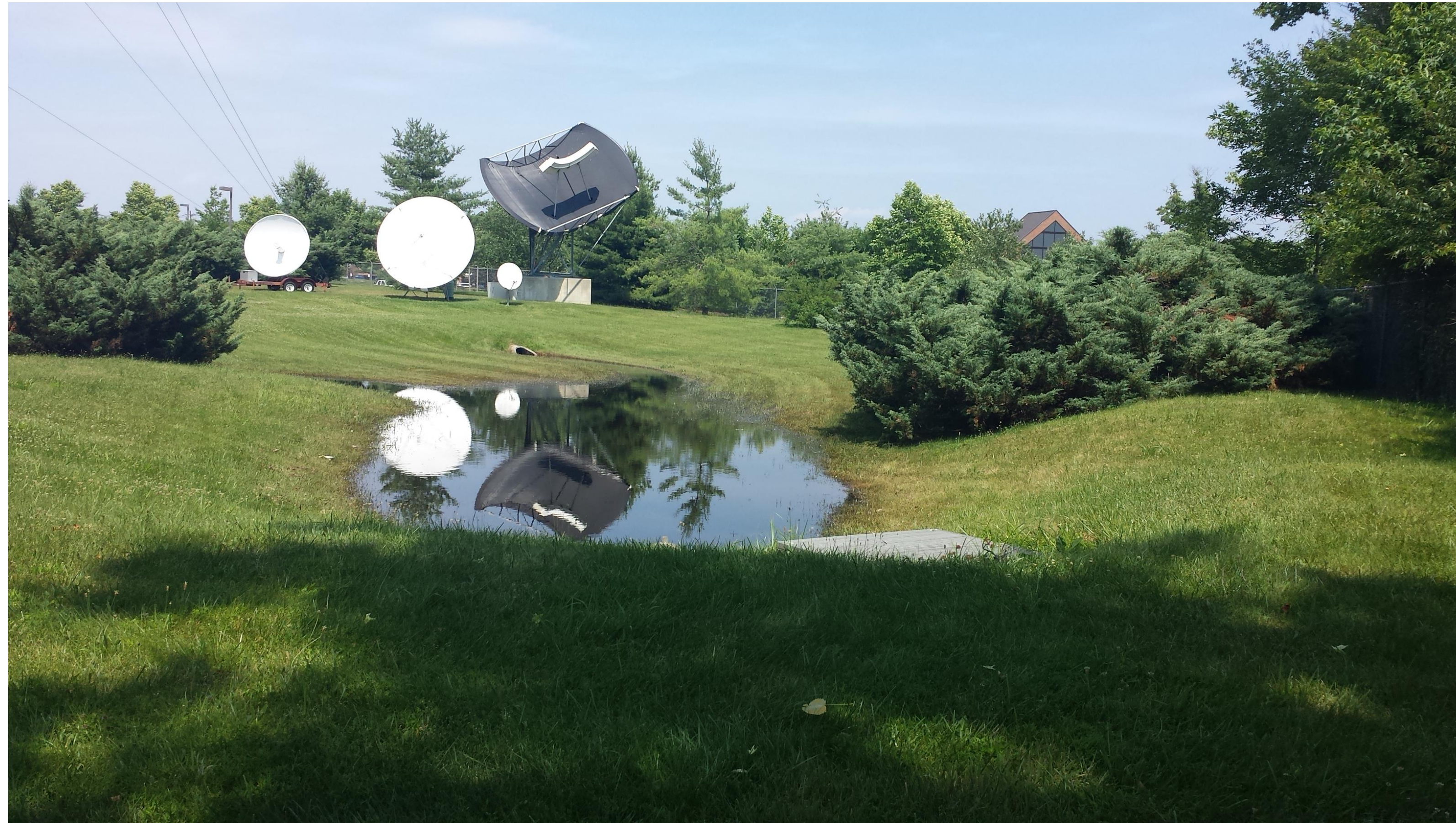
Overview of basin
