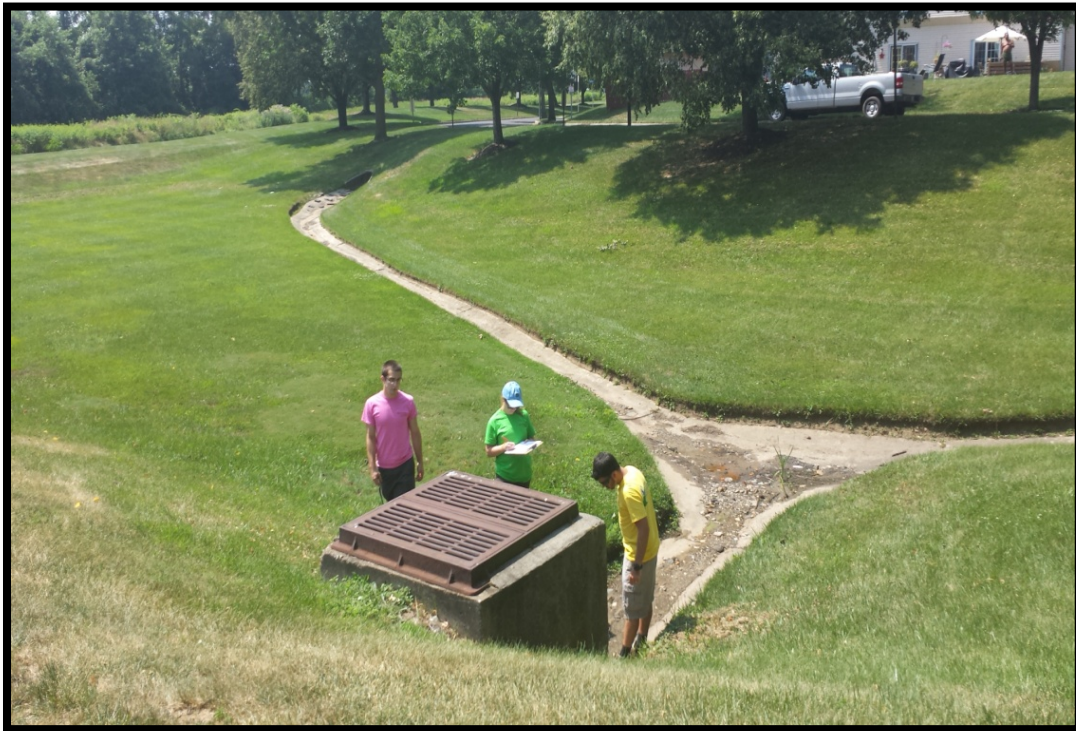
Student interns measure outlet structure at Ravenscoft basin
