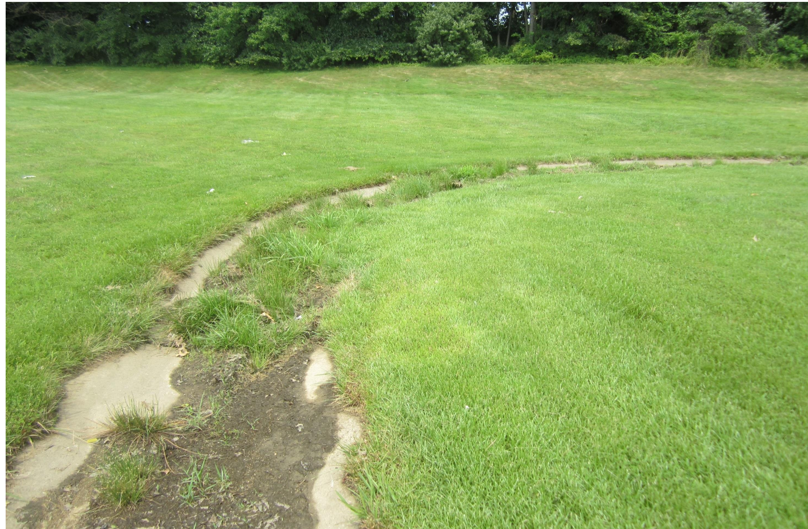
Sediment in low flow channel
