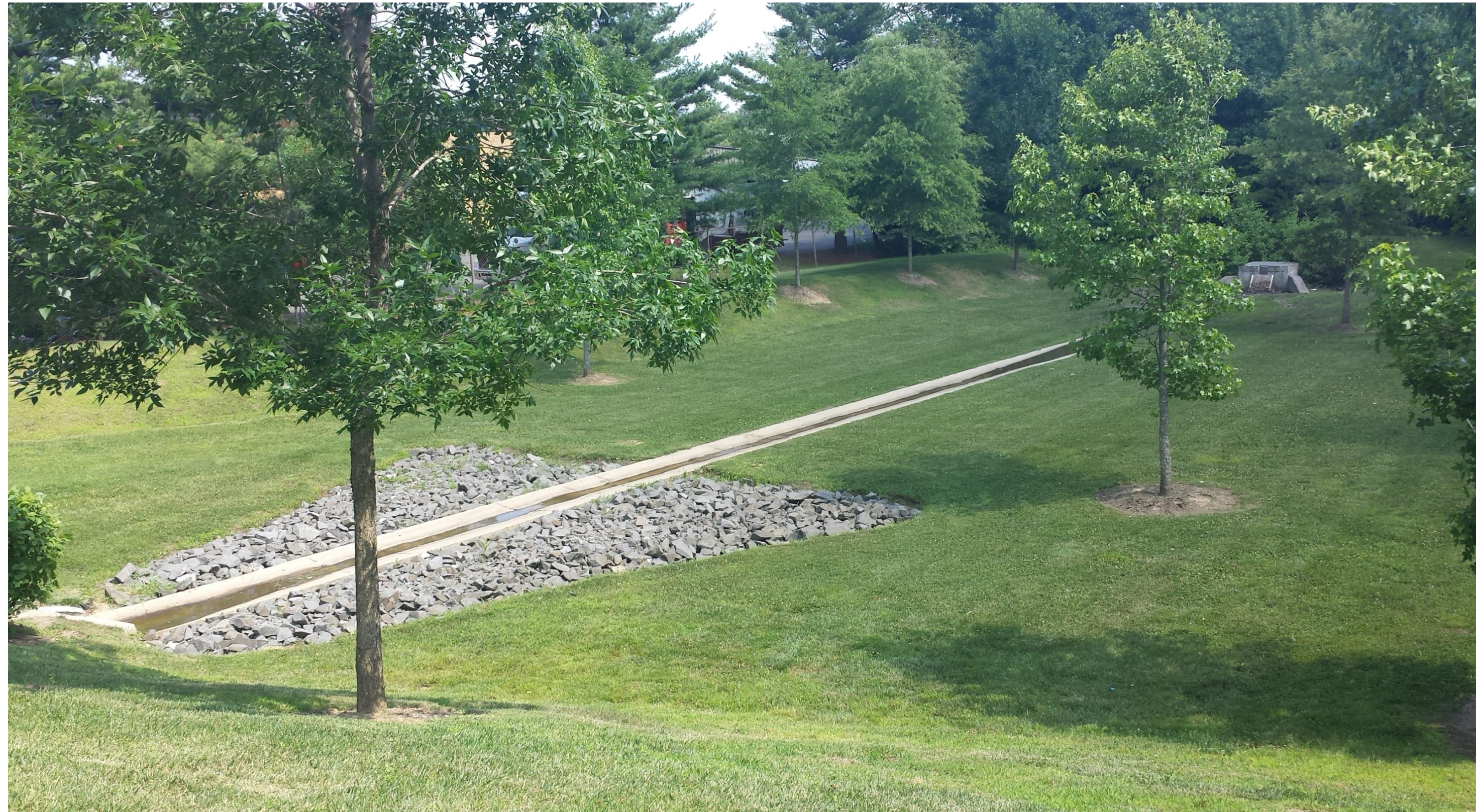
Overview of basin
